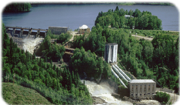
Canadian Hydroelectric Facility in the Great Lakes Basin
